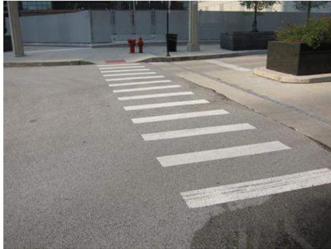
**Figure 19. High Visibility Crosswalk** (source: FHWA)
